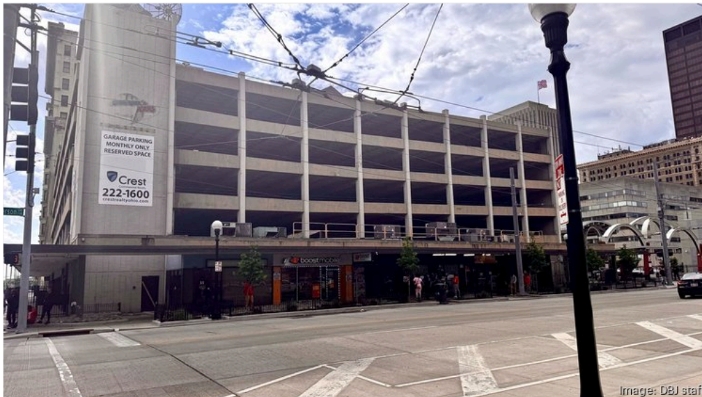
Air City Garage at the corner of E. Fourth Street and S. Jefferson Street
